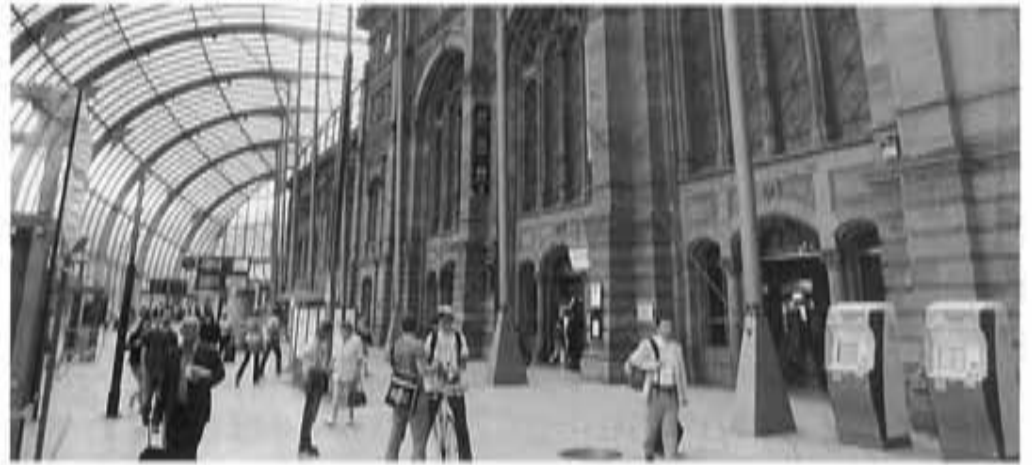
▼ Revamped railway station, Strasbourg
